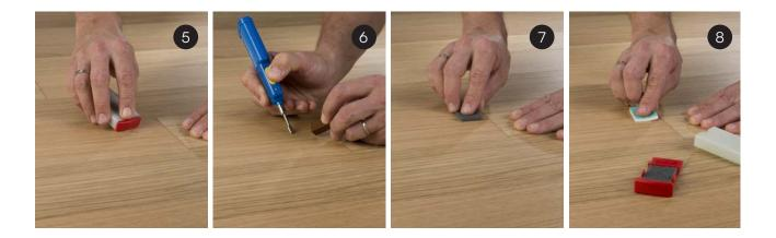
**CLEANING:** Use the cleaning comb to clean the planer grooves. Just wipe off melting knife with a cloth after use.
